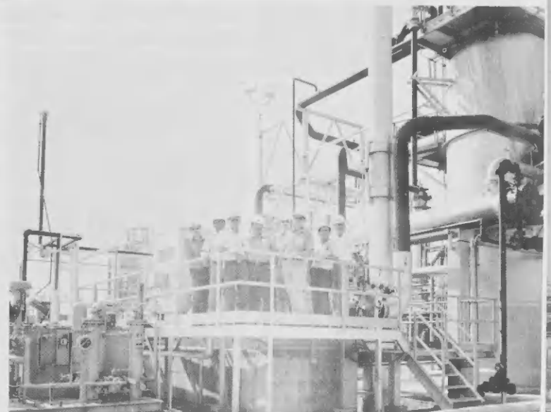
Some of the Mechanical and TOA personnel involved in the G2AR startup are from left to right: Donny Henriquez (EIS), Al Connor (Rotating Equipment), B. Lofflo and Candy Koolman (Mechanical), Mickey Eckert (EIS), J. Higginbotham (TOA), Ev. Beaujon (Process Foreman), Ricardo Gee (Electrical) and Z. Johnson (TOA).
